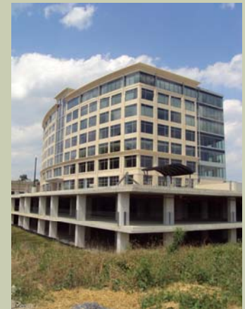
Office Building "E"
